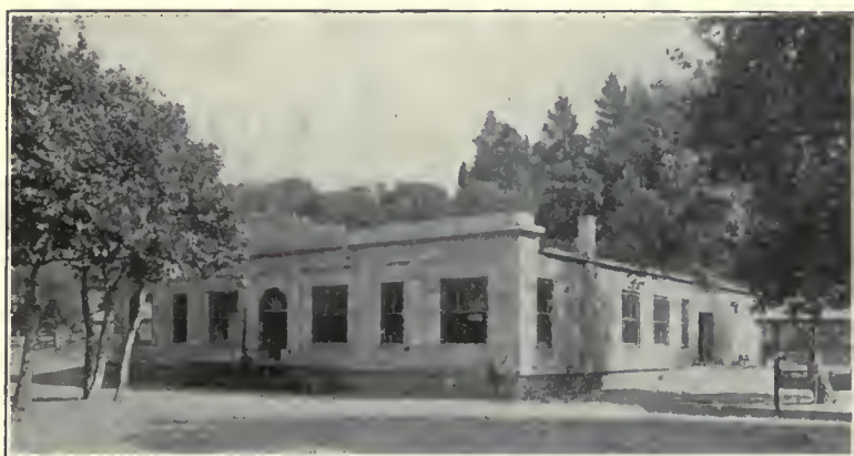
New Cresta Blanca Bottling Cellars. Concrete, 80x100 ft.
